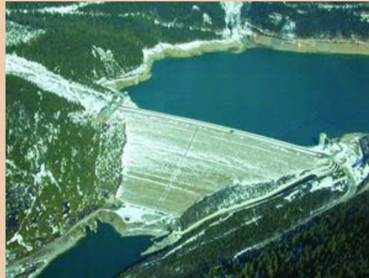
Mica Dam built in 1973
